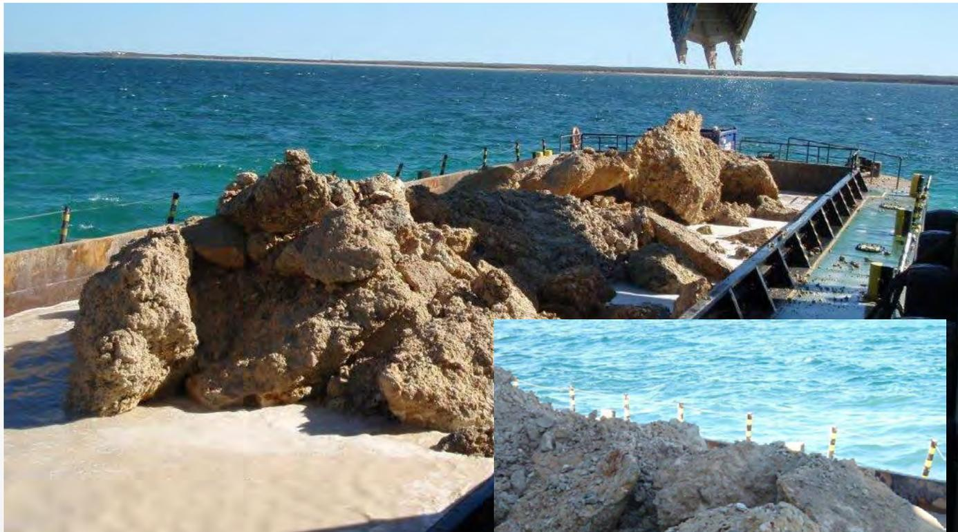
Direct dredging of the Coastal limestone by the newly built jumbo backhoe Baldur was successful. The top of the unit was expected to be stronger (calcrete / caprock), but the thickness of this caprock was higher than expected.....
