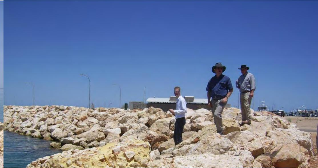
The breakwater consists of large armourstone blocks, locally brecciated and fractured.
