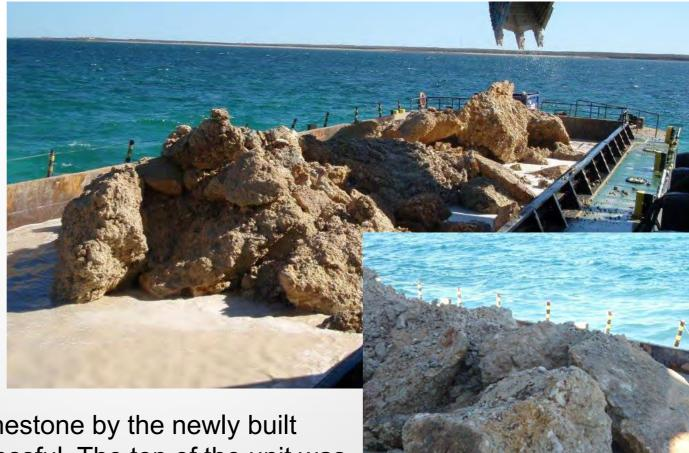
Direct dredging of the Coastal limestone by the newly built jumbo backhoe Baldur was successful. The top of the unit was expected to be stronger (calcrete / caprock), but the thickness of this caprock was higher than expected.....
