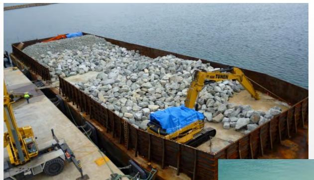
Often loads with multiple gradings and equipment – lowering barge capacity
