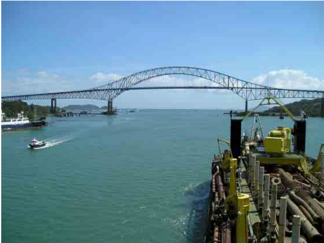
Dredging under the bridge of the America's
