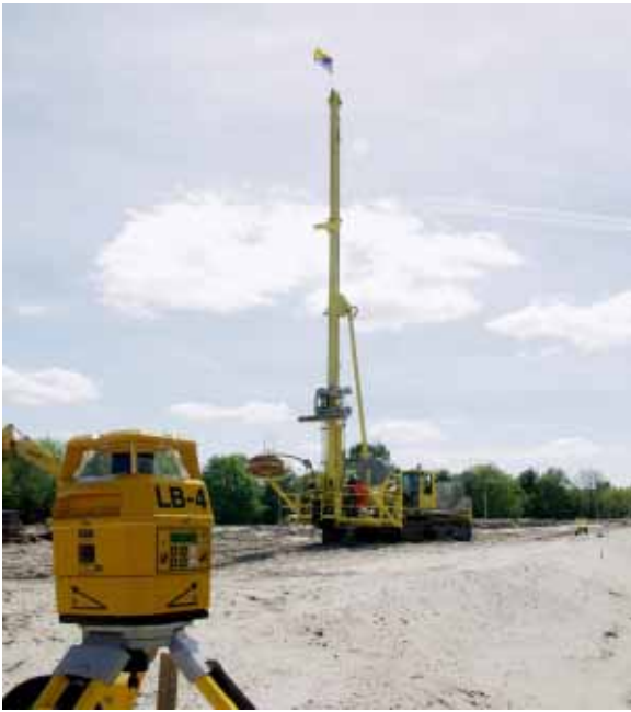
Figure 3: BeauDrain installation
