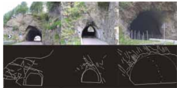
Figure 10: Overbreak decreases with decreasing bedding thickness. Again an example demonstrating that the RMR is not directly related to the overbreak. Passeirertal (I).
