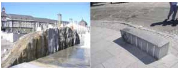
Figure 4: Evidence of accurate blasting: half pipes in LST. Place St Lambert, Liège.
