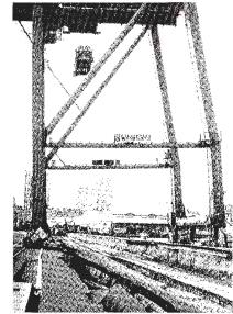
Figure 2 Destruction of service area due to failure of quay wall.
