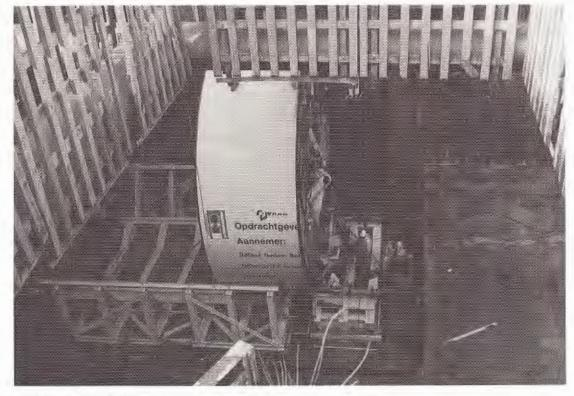
Figure 9 Part of the TBM set up in the sourt pit
