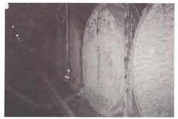
Figure 8 View along the longitudinal pipe with concrete filled transversal pipes at the right side.
