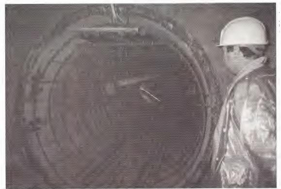
Figure 7 Transversal pipe (Ø 1.90m) with reinforcement and filling tube for concrete (centre).
