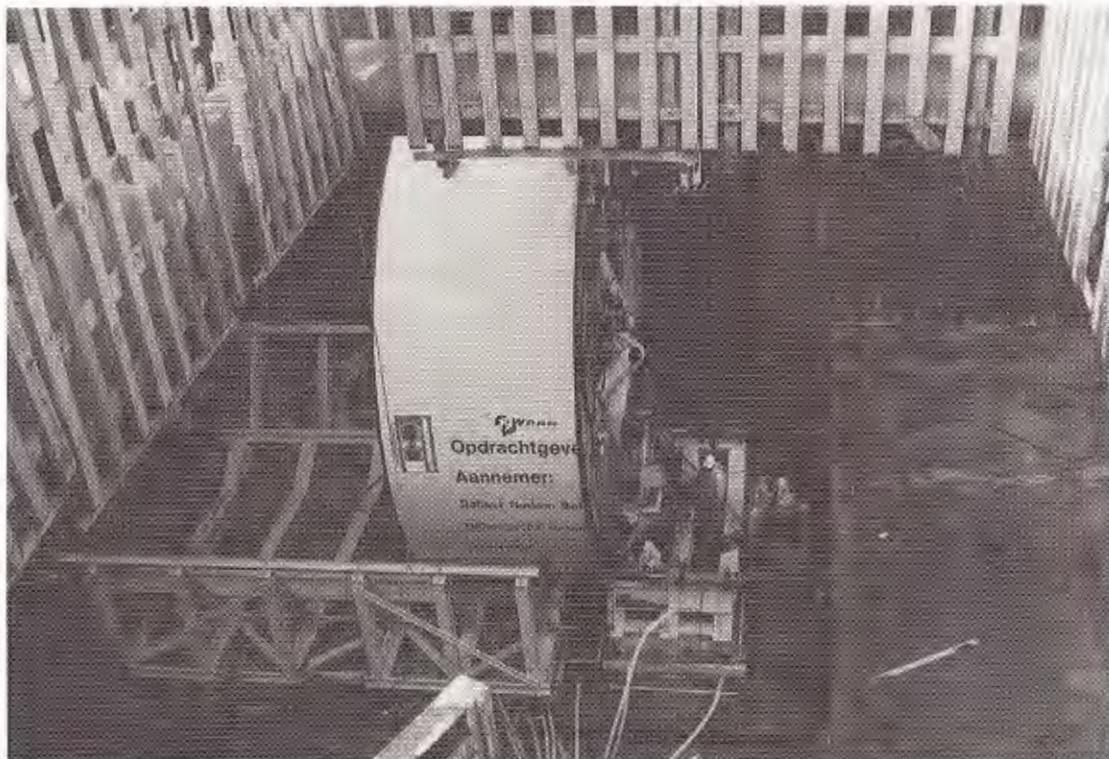
Figure 9 Part of the TBM set up in the start pit
