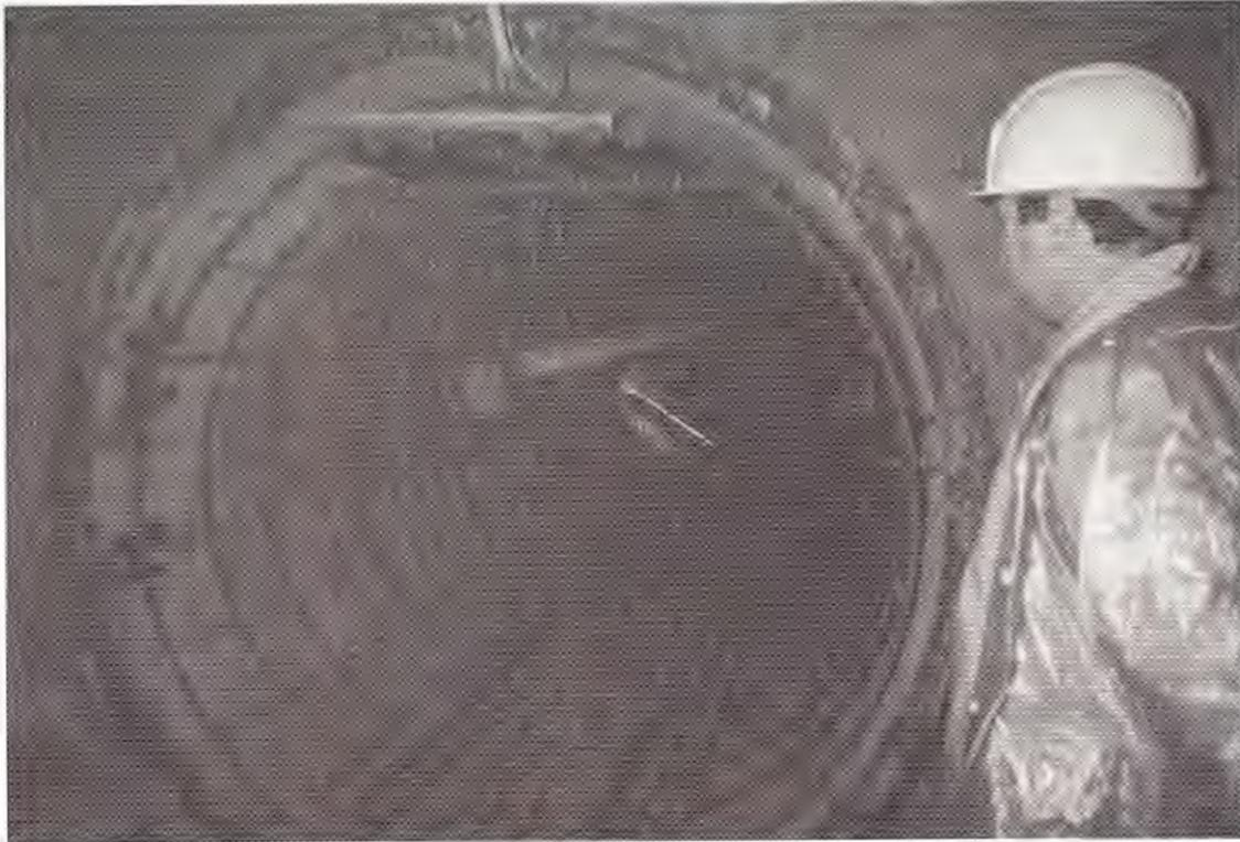
*Figure 7 Transversal pipe ( $\varnothing$  1.90m) with reinforcement and filling tube for concrete (centre).*
