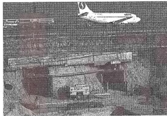
**Figure 4** Undercutting beneath a Sub-terrain Roof Plate at Section B1 (looking S to N); Two Galleries are in use (Photo: centrale studiedienst de lijn).
