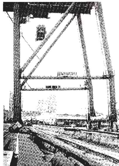
Figure 2 Destruction of service area due to failure of quay wall.
