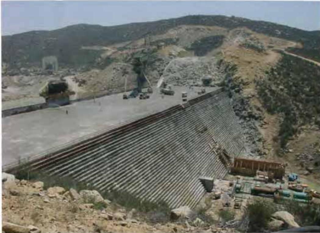
Roller-compacted concrete Olivenhain Dam in San Diego, CA.
