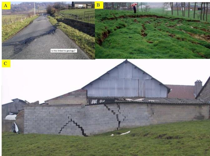
Figure 2. Examples of failures caused by slope movement in the Land of the hills / Flemish Ardennes. A: Local road damaged by slow slope movement. B: Fissures in a pasture caused by slope movement (reproduced with permission of Vanhulle, 2005). C: Farm house located on a hill damaged by slow slope movement analysed by the authors in 2002.
