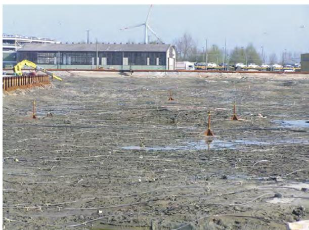
Figure 5 BeauDrain-S system after lowering of water table and connection of HDPE tubes.
