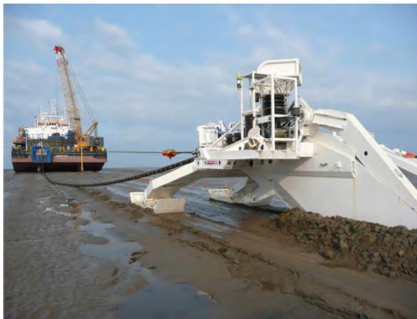
Figure 4 Cable burial using a cable plough.
