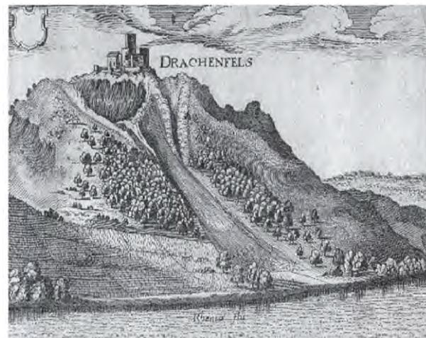
Figure 2 On this copper gravure of the Drachenfels, a volcanic neck of trachyte, the chute used to slide building stone blocks downslope from the quarry below the castle is clearly visible.
