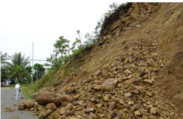
**Figure 1** Rock slope failure on road cut slope due to stress changes and weathering.
