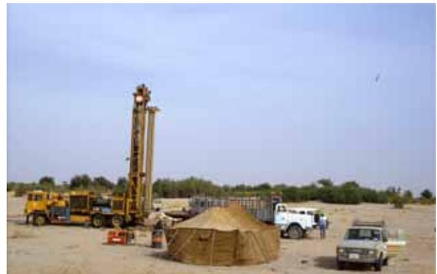
Fig. 5 Exploratory drilling of aquifers in Marib region.
