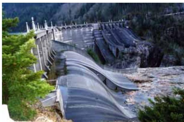
Fig. 15 *View of the Diablo Dam spillways resting on metamorphic rocks of the Skagit Gneiss Complex* (source: author's photo).
