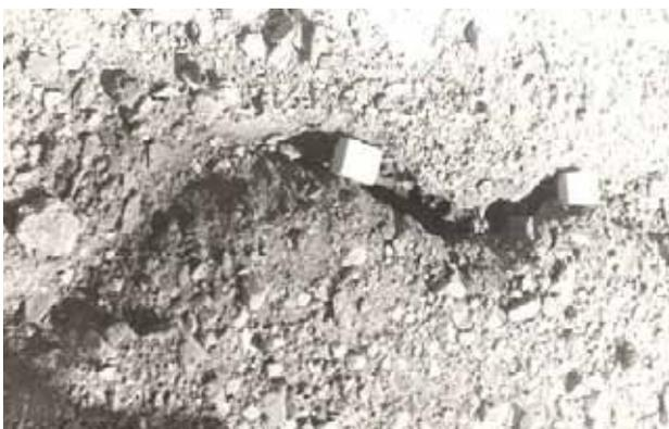
Fig. 4 Transversal crack created on dam axis.
