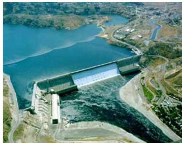
*Fig. 8 Grand Coulee Dam, with Right and Left Powerplants at both sides of the spillway and Third Powerhouse and Forebay Dam at the left side (source: U.S. Bureau of Reclamation).*
