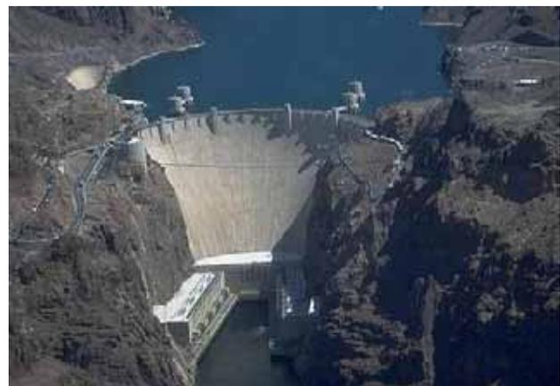
Fig. 4 Aerial photo of Hoover Dam with the U-shaped power plant in front and Lake Mead in the back (source: photo.net/photo/pcd2882/hoover-dam-aerial-91.4.jpg).
