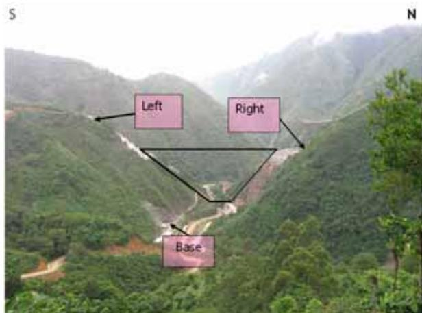
Fig. 2 Dam site looking downstream with sketch of dam and placement of accelerographs.
