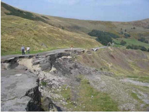
Road damage on the Mam Tor landslide.
