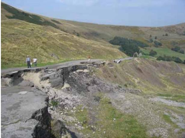
Road damage on the Mam Tor landslide.
