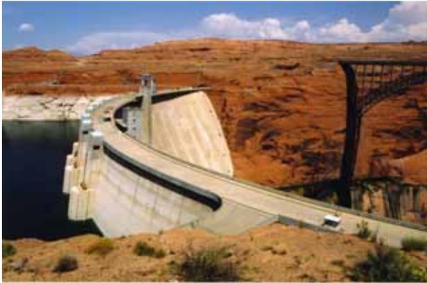
Fig. 2 Glen Canyon Dam and Bridge (note the white band on the Navajo Sandstone, result of the low level of the reservoir behind the dam) (source: author's photo).
