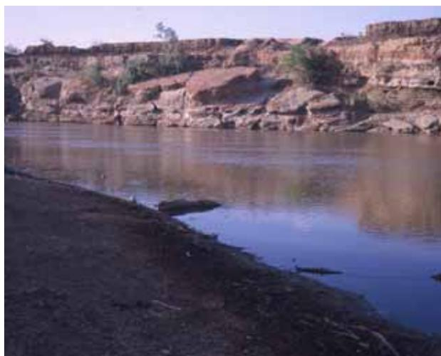
Photo 9 Collapse of a slope along the river bank in gypsiferous rock. Dissolution is clearly an element determining the stability of the slopes.
