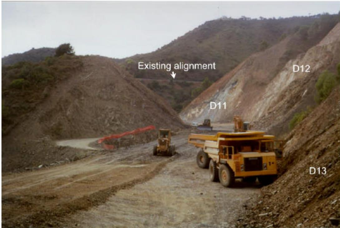
*Figure 3. Construction work going on at slopes D11, D12 and D13; existing road alignment just above center*
