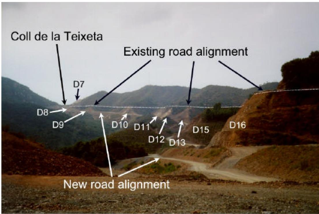
**Figure 2.** A view from slope D17, close to Coll Negre, towards Coll de la Teixeta with the visible slopes indicated
