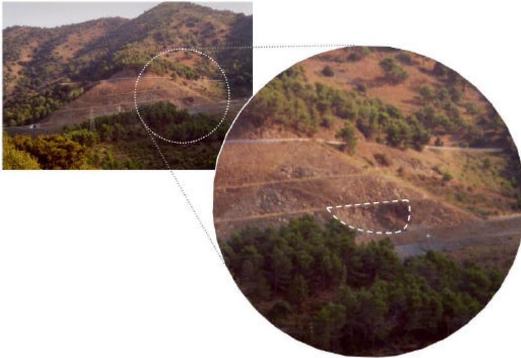
*Figure 6. Slope D16, looking north – the scar of a rotational slide in the lower right part*
