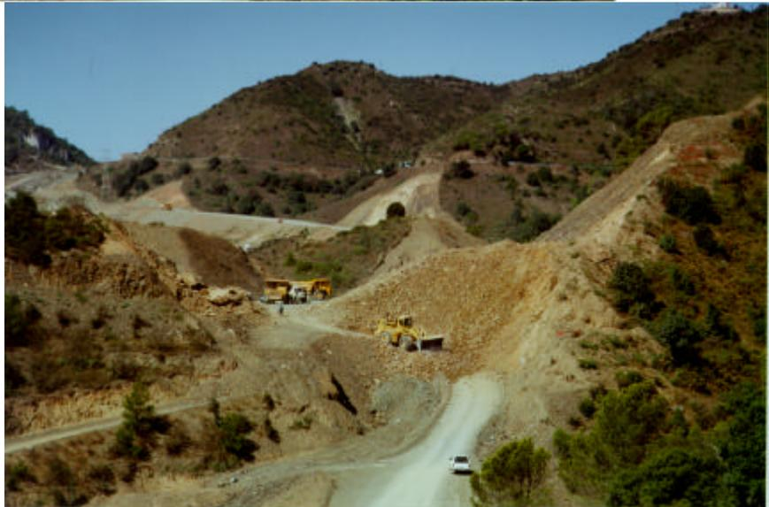
*Figure 5. Blasting of the lower part of slope D13*
