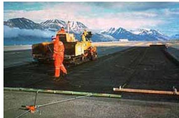
**Figure 3** Installation of asphalt reinforcement grids (source: [www.huesker.de](http://www.huesker.de)).
