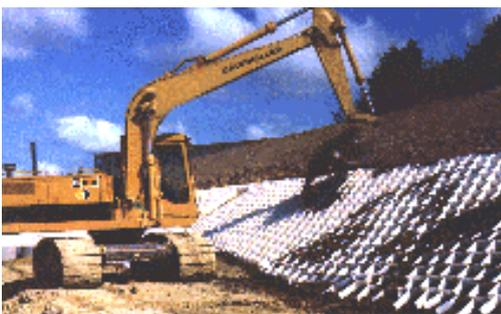
**Figure 2** Installation of erosion protection
