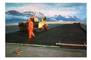
Figure 3 Installation of asphalt reinforcement grids (source: <u>www.huesker.de</u>).
