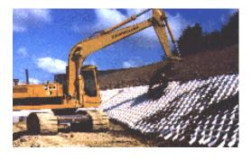
Figure 2 Installation of erosion protection (source: www.geosynthetics.nonwovens.akzonobel.com/).
