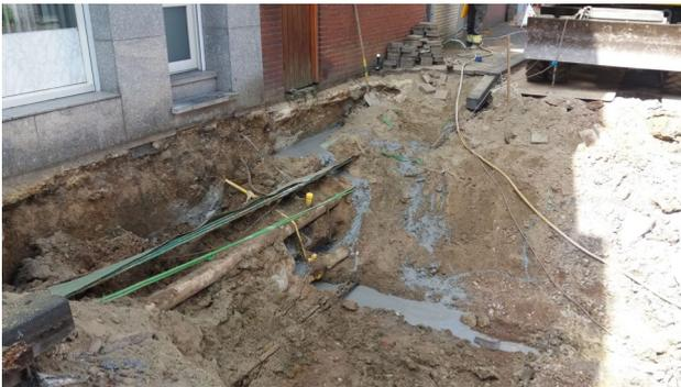
Figure 3 Filled-up voids in front of residential building at the sinkhole shaft DOM 37
