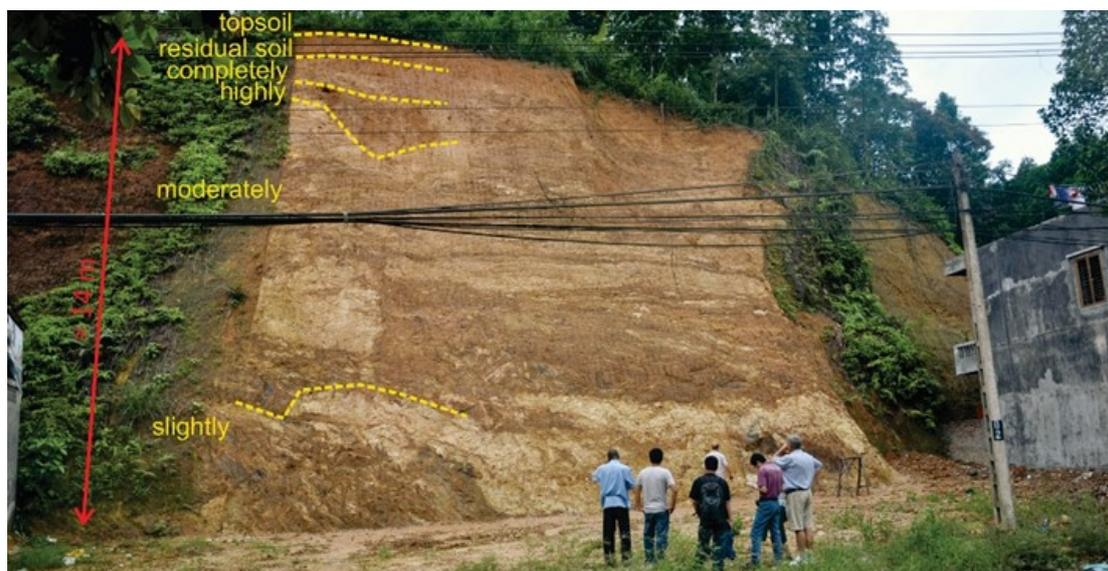
Figure 1 Deep mainly chemical weathering in a cut slope in gneiss and schist in a tropical climate (weathering grades follow ISO 14689-1:2017 (2017) for rock masses) (Yên Bái City, Vietnam; photo courtesy D. Alkema, 2010)
