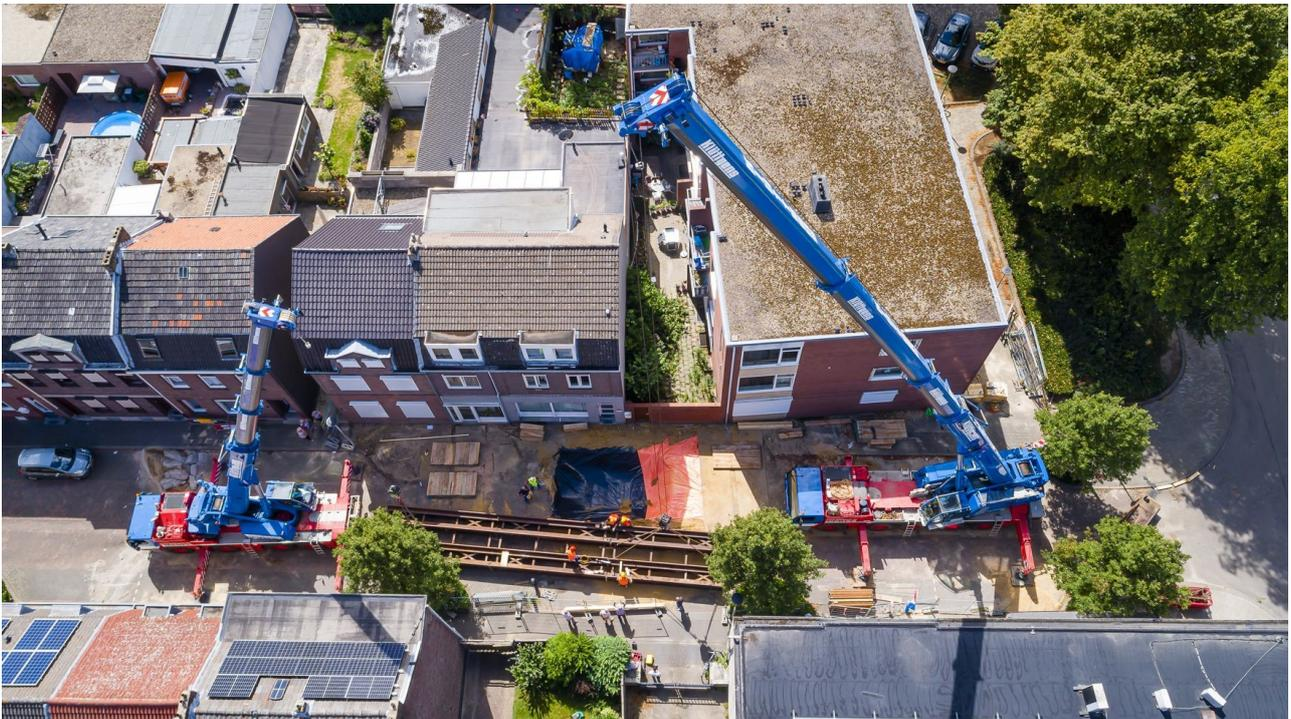
Figure 5 Installing the 18 m-steel-bridge above shaft DOM 37 (Picture by GbE, Grundbau Essen GmbH)
