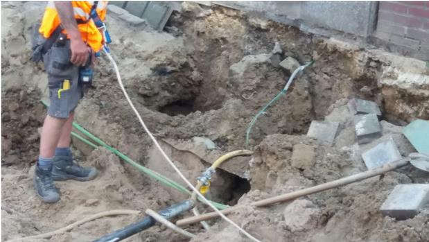
Figure 2 Tube-shaped voids in front of the residential building at the sinkhole shaft DOM 37
