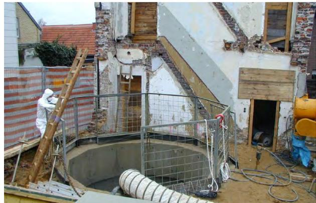
*Shaft remediation by refilling with cohesive material (including clay).*
